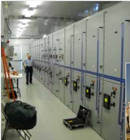
Prime Power control & Distribution building package for US military facility in the Middle East. Interior view of switchgear, rated 2000A @11kv 50Hz.
